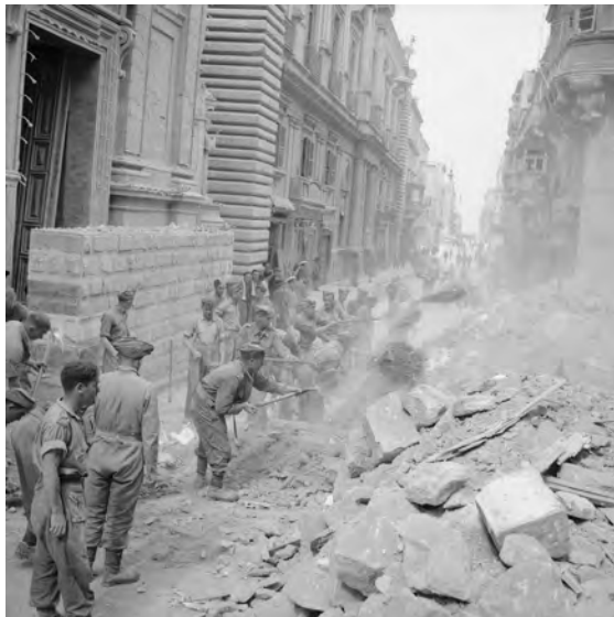
Bomb damage to the streets of Valletta in 1942, illustrating the intensity of bombardment the Island suffered and the scale of the engineering tasks the Royal Engineers faced By Lieutenant H E Cook, War Office official photographer
