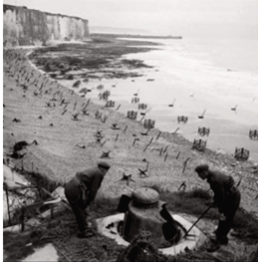
Heavily fortified stretch of the Normandy coast.
