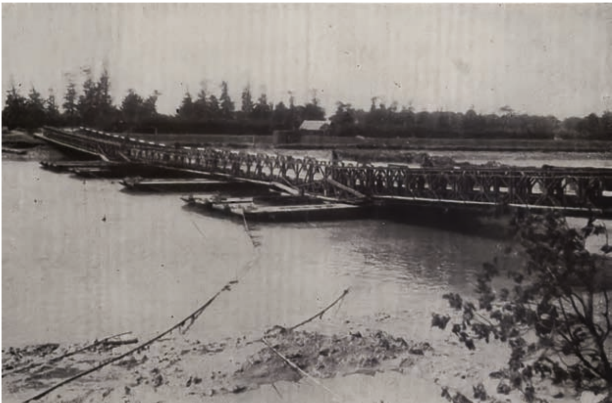
YORK 1 class bridge with boom in foreground
