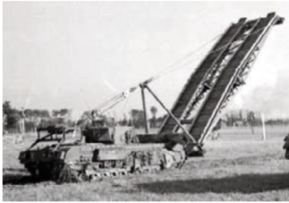
Churchill AVRE Mk III with Small Box Girder (SBG) Bridge. It could cross a 9 m gap or surmount a seawall up to 3.6 m high.
