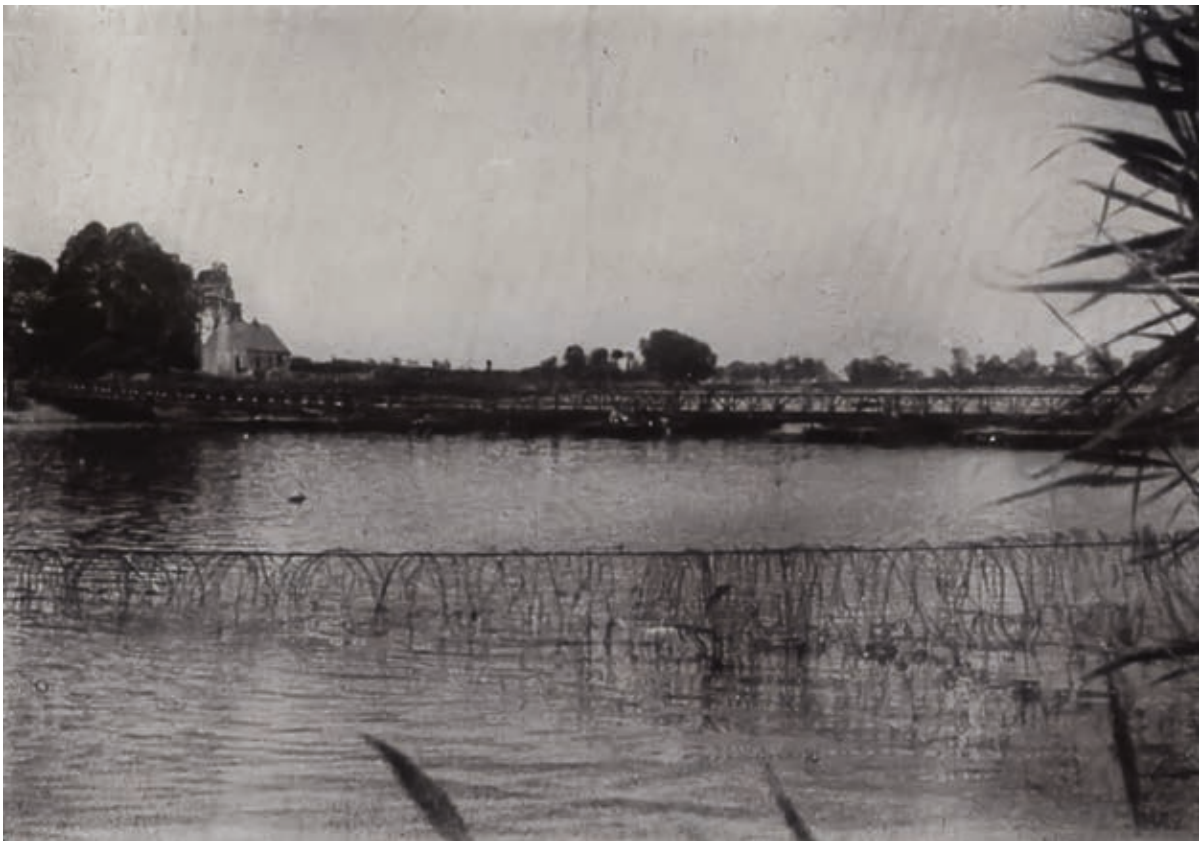
YORK 1 class bridge with boom in foreground
