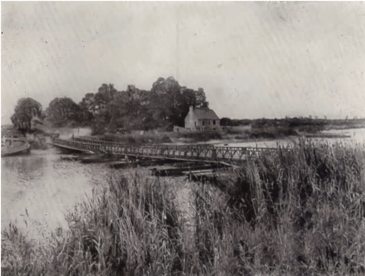
YORK 1 class 40 Bailey pontoon bridge over CAEN Canal (view looking West)
