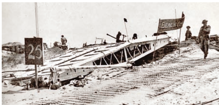
SBG Bridge over ditch at head of Beach 15
