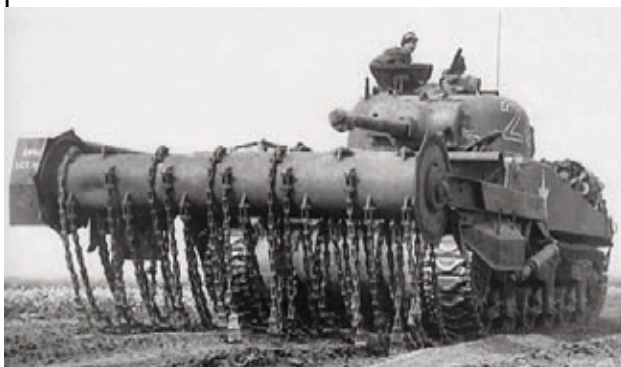
Sherman Mk IV Flail ('Crab'). The flail was driven by the tank's engine and would cross a minefield at about 1½ mph, clearing a path 2.7 m wide.
